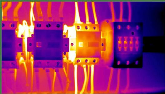
**Electrical infrared Inspection**
